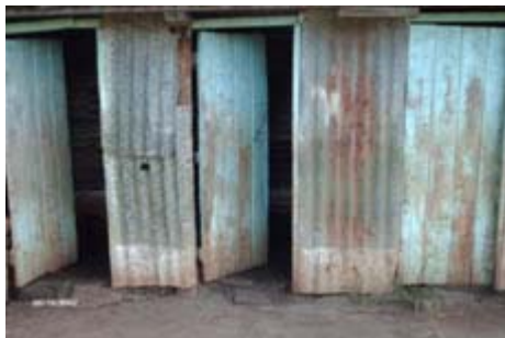
A typical primitive toilet facility at the early stages of the kibbutz
